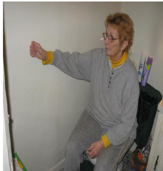
Pre-modification: No grab bar to assist with transfers
