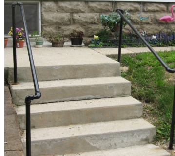
Post-modification Double handrails on stairwell
