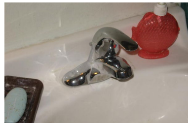
Post-modification Lever handle installed for easier use
