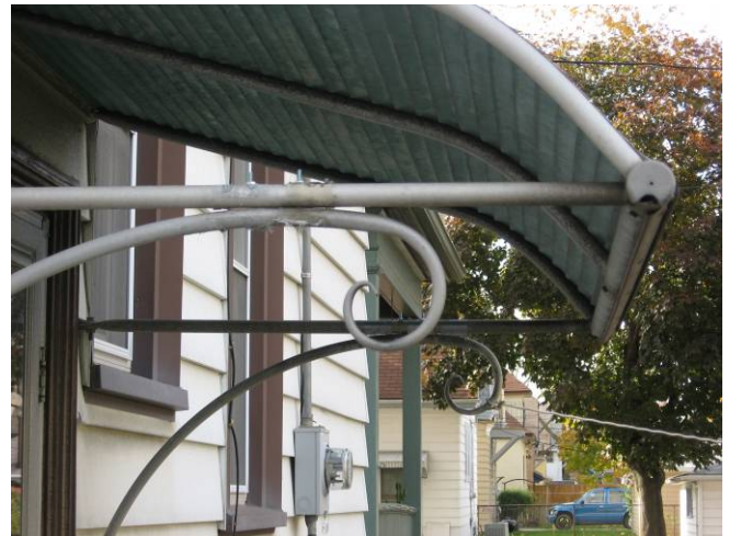
Image 9 After: Awning repaired with bolts
