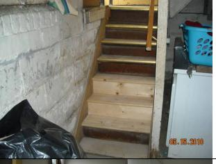
The basement stairs in this home needed to be replaced. The picture on the left reveals several broken steps. The stairs pictured on the left also lack a railing. The picture on the right reveals the replaced stairs and addition of a railing.
